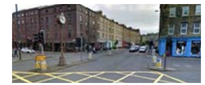
TOLLCROSS JUNCTION AT CORNER OF BROUGHAM STREET
