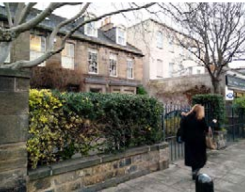
3: Boring: Whilst attractive, housing is often withdrawn from the street and has a garden or fences facing the street but with little activity.
