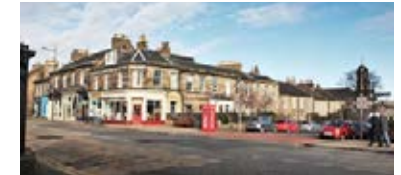
PORTOBELLO HIGH ST AT JUNCTION WITH BELLFIELD ST
