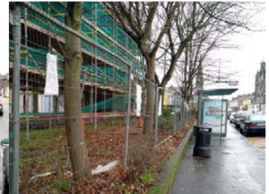
4: Construction site facing the street.
